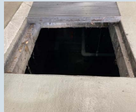
Rainwater Inlet Installed at the Nagoya Head Office Building Parking Lot
