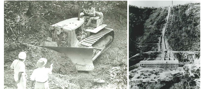
Construction Scene of the Baluchaung No.2 Hydropower Plant
