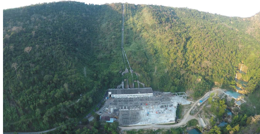
View of the Baluchaung No.2 Hydropower Plant
