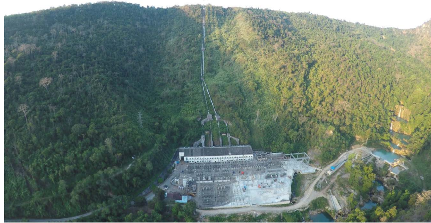
View of the Baluchaung No.2 Hydropower Plant
